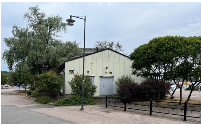
Figur 9 – Pumpstation PB7 i Oskarshamn
